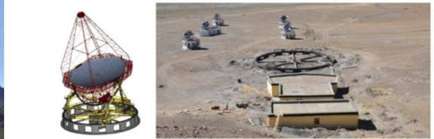
Left: The MACE telescope design. Right: Civil work at Hanle: MACE foundation and control room.
